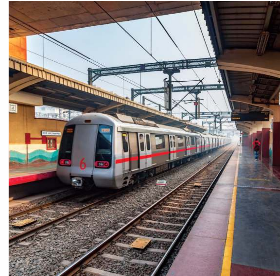
Upcoming Metro connecting Hinjawadi to Shivaji Nagar
