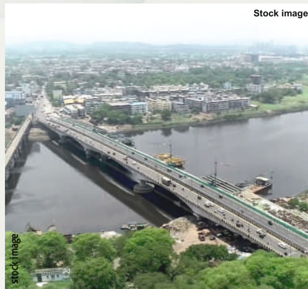
Ready Durgadi Bridge
