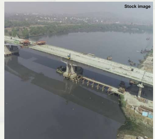
Dombivali Mumbai Bridge (Under Construction)
