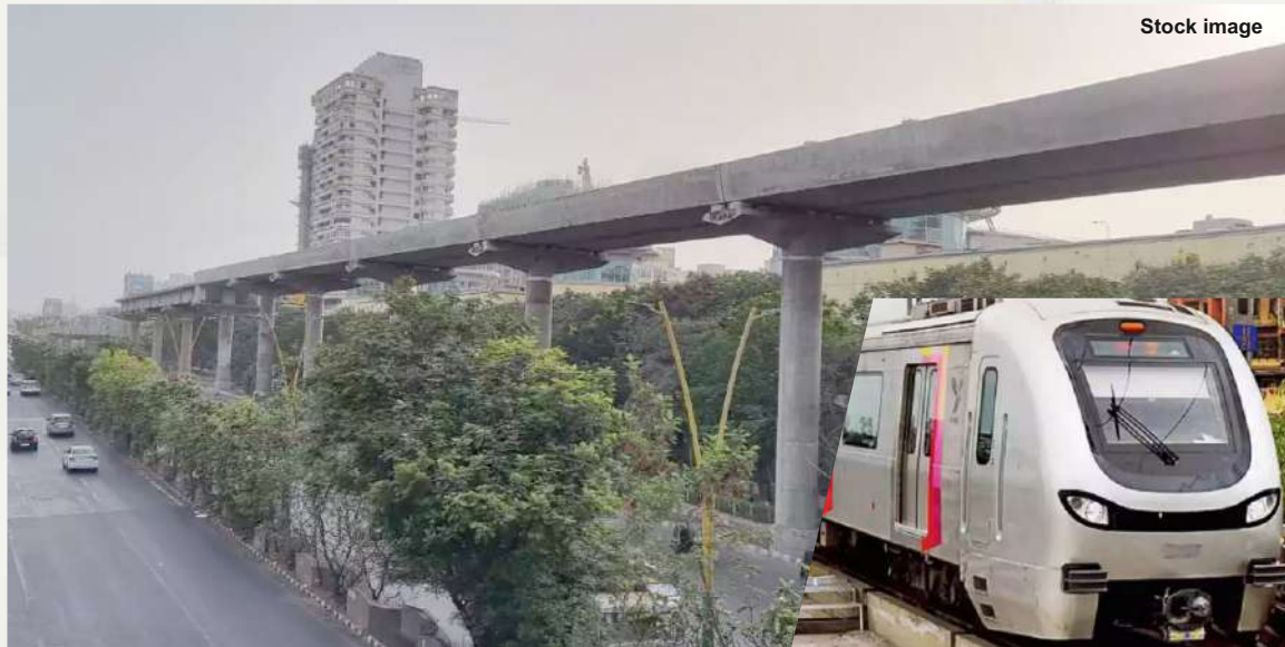
Work In Progress Metro Line 5
