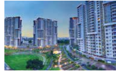
Greenage Hosur Main Road, Bengaluru
