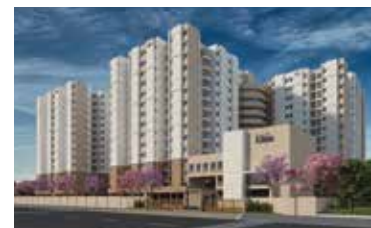
Ashraya Mysore Road, Bidadi, Ramanagara
