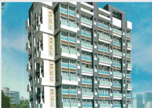
Durga Nagar (E Wing Completed, F Wing Ongoing)
