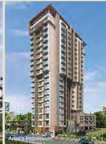
CREST Andher (W)
