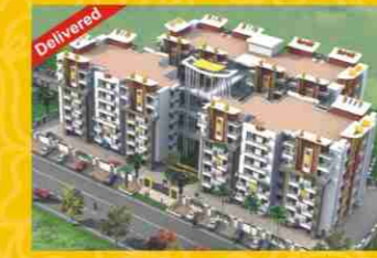
Rudra Towers Sunderpur, Varanasi
