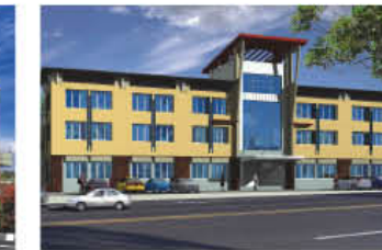
The Mall Kanpur
