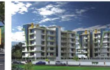
Rudra Twin Towers New Berry Road, Lucknow
