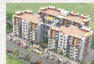
Rudra Towers Sunderpur, Varanasi
