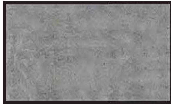
Exposed Concrete Finish
