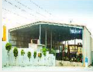
BCC PRECAST PLANT
