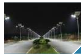
INTERNAL RCC ROAD WITH STREET LIGHT
