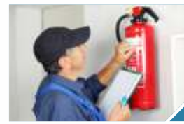
FIRE SAFETY SYSTEM
