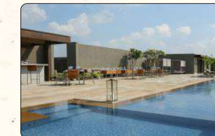
ROOF TOP SWIMMING POOL
