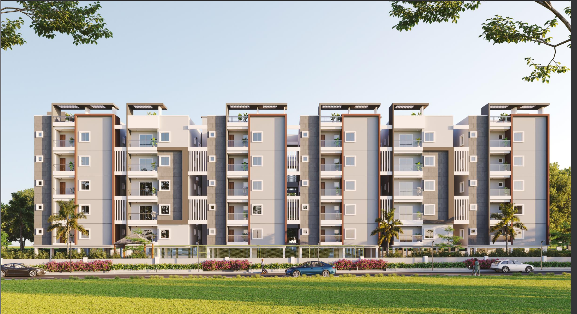
BLOCK-C FRONT VIEW
