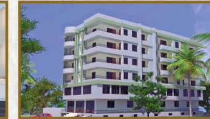
EXCEL TOWER NADESAR
