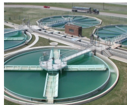
SEWAGE TREATMENT PLANT
