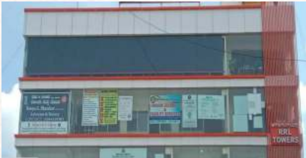
RRL Tower - Completed
