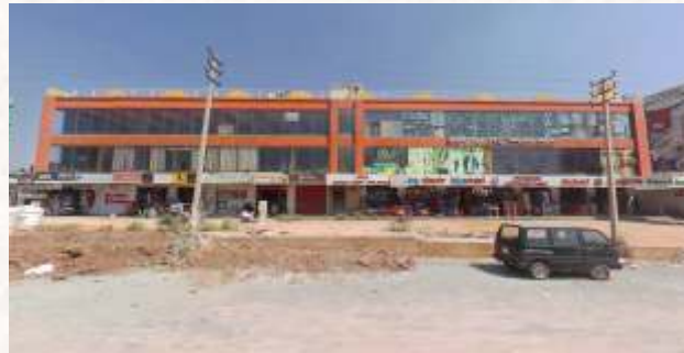
RRL Complex - Completed
