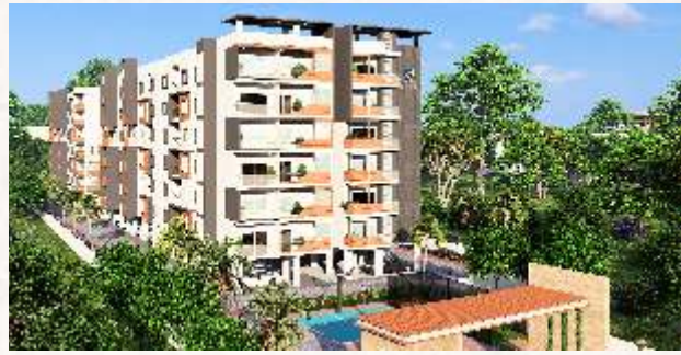
RRL Palacio - Ongoing
