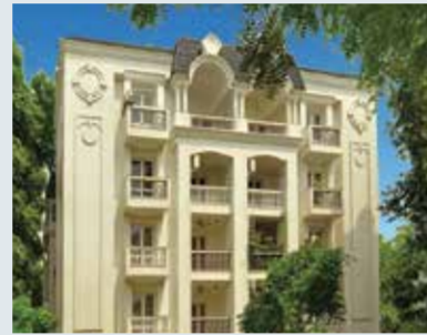
SHALIMAR ROYALE MALL AVENUE
