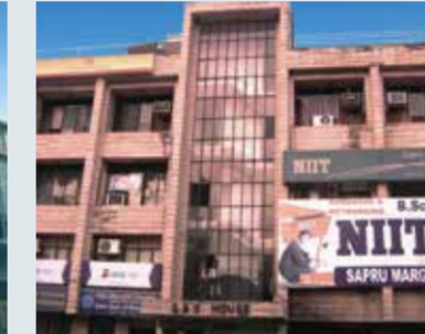
SAS HOUSE SAPRU MARG
