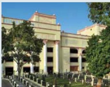
MULTILEVEL PARKING HAZRATGANJ
