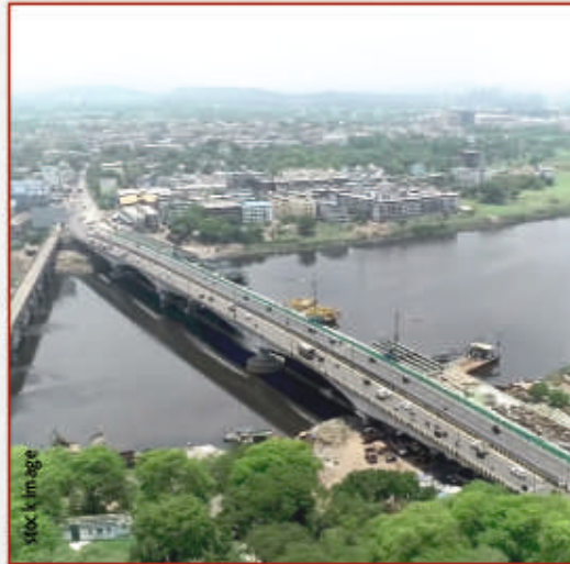
Ready Durgadi Bridge
