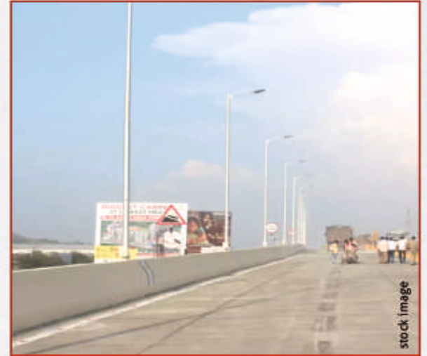
8 Lane Highway (Work in Progress)
