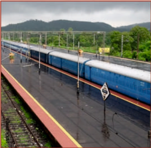
Thane - Virar Railway Work In Progress
