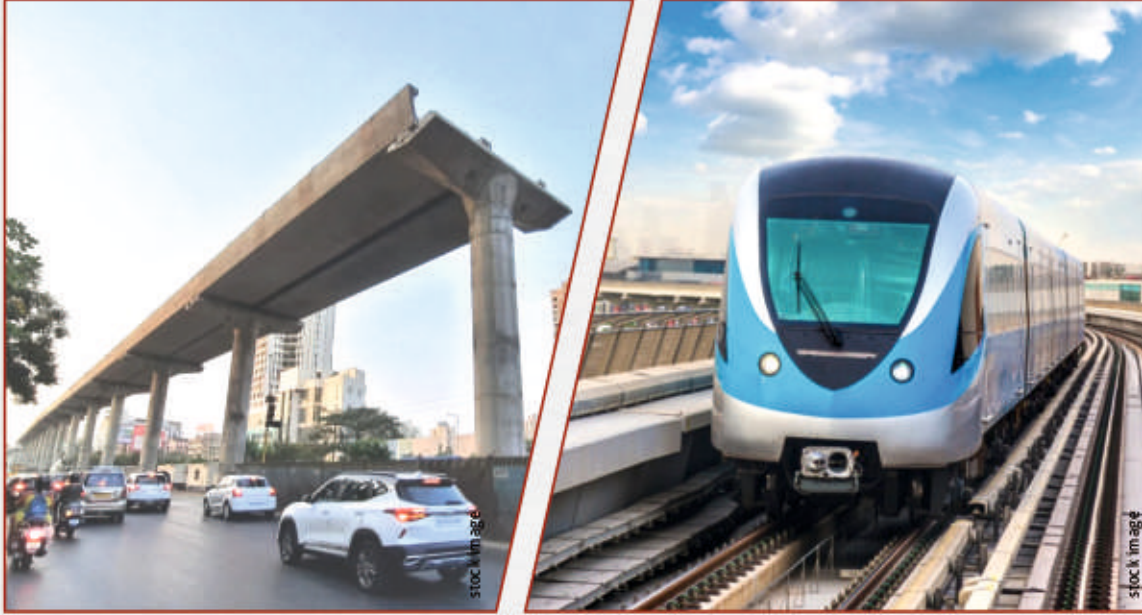
Work In Progress Metro Line 5
