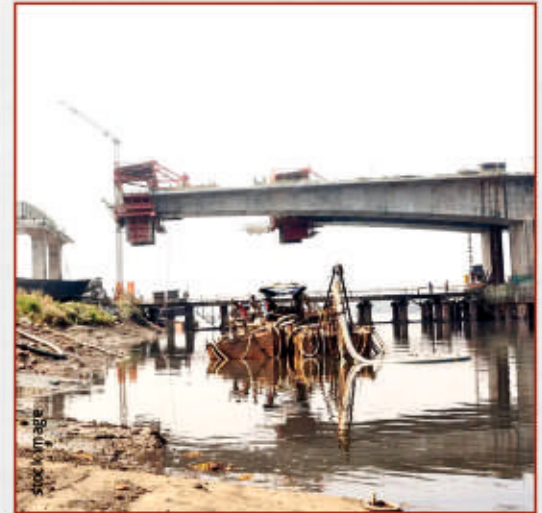
Dombivli Mankoli Bridge (Under Construction)
