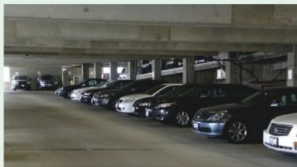
Covered Car Parking
