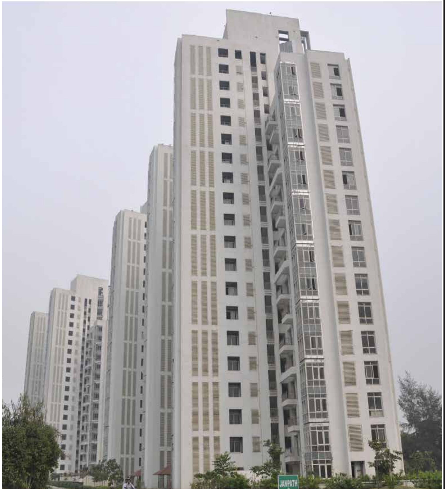
Actual Picture of Moon Court Apartments
