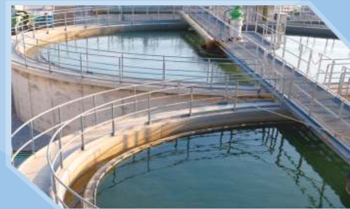
SEWAGE TREATMENT PLANT
