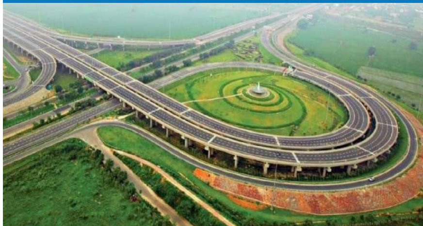
MUMBAI - DELHI EXPRESSWAY
