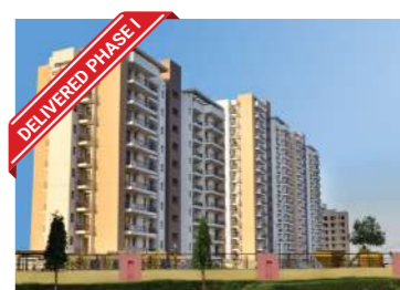
SECTOR 37C, GURGAON DWARKA EXPRESSWAY
