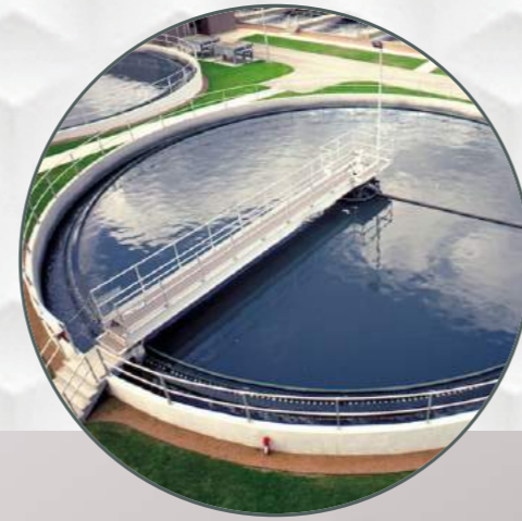
Sewerage Treatment Plant (STP)
