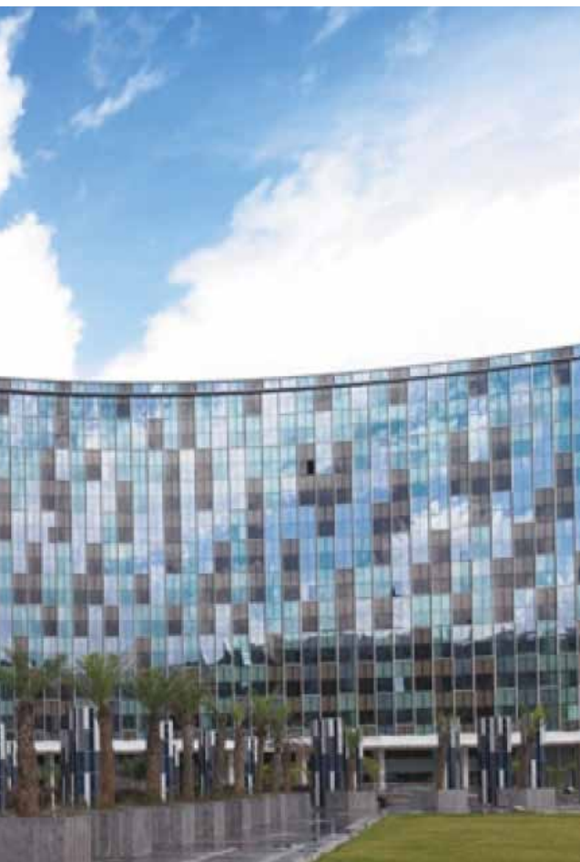
Facade view of an IT park building
