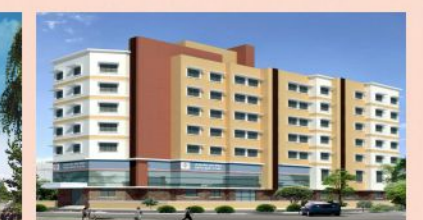
HOSTEL BUILDING - KURLA
